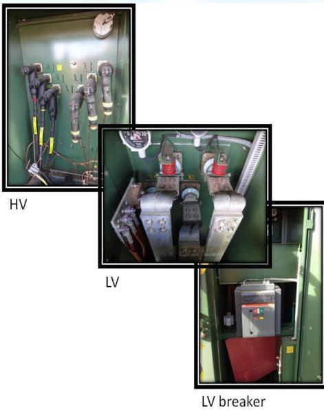
High voltage elbows, arresters, low voltage configurations and terminations, wired accessory packages, and low voltage breakers are but a few of the possible items which may be unique to the transformers supplied for the project.
