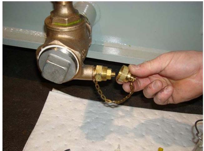
Remove protective cap on sampler cap to expose the fitting.
