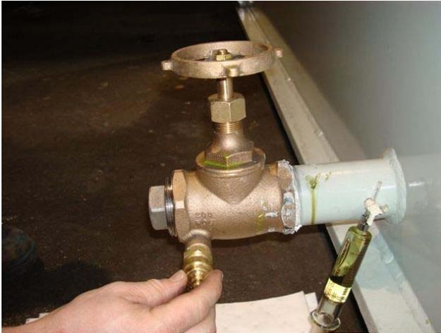
Confirm the valve handle closed (clockwise) and the sampler protective cap is tight
