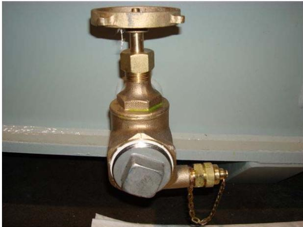
Locate lower drain valve with sampler fitting. Check valve handle and be sure it is closed
