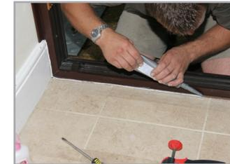
A blunt wood chisel was used to poke the tube into place.
