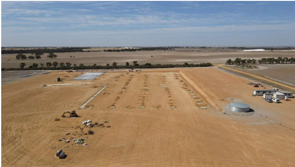
Figure 1. Aerial view of the building work commenced at Wickepin
