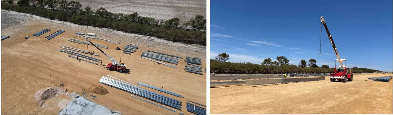
Figure 2. Structural steel arriving onsite in Wickepin
