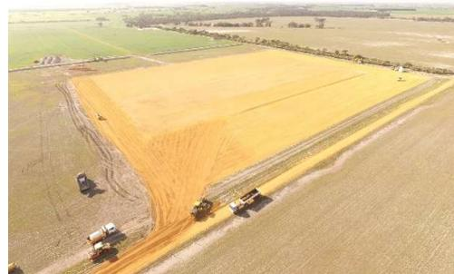
**Figures 1 and 2:** Plant preparation earthworks completed on site at Wickepin
