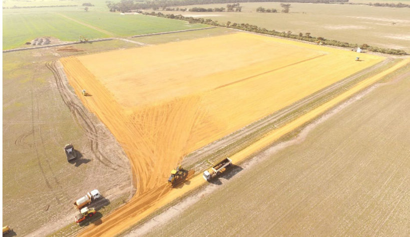
Figure 2: Wickepin Stage 1 earthworks in construction
