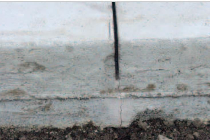
When drying shrinkage and the resulting cracking occur shortly after placement (while the concrete is still soft, or “plastic”), we use the terms *plastic shrinkage* and *plastic shrinkage cracking*. The difference between plastic and drying shrinkage is therefore only the condition of the concrete when the drying, shrinkage, and cracking occur. And the key to controlling them both is to find ways to reduce the rate of drying of the concrete.
