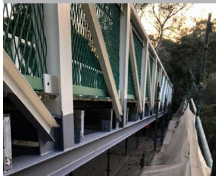
Final coat to handrails and intermediate coat to underside with containment erected to capture any falling debris
