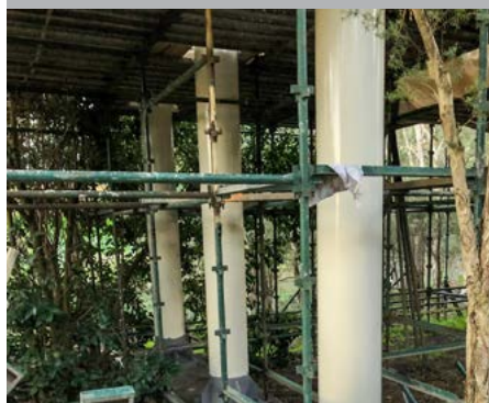
Bridge piers were cleaned and coated with a three-part protective coating system
