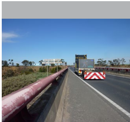
Metalwork on the outbound lane of the bridge showing signs of deterioration
