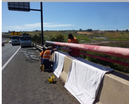
Metalwork cleaned and, where required, spot treated and primed, in preparation for the protective coating
