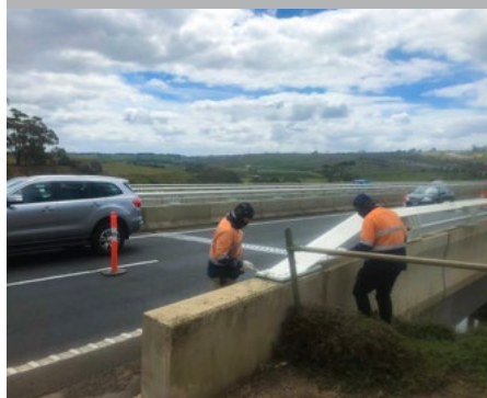
Workers applying the final coat to the bridge metalwork
