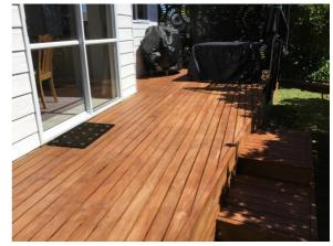
The deck on the southern side of the building is of timber slatted construction and is attached directly to the building. It is framed with timber joists and has timber posts.
