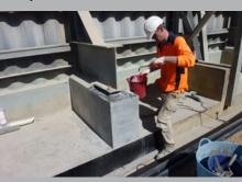
Once repairs were complete all plinths were ground back to a flat surface and cleaned of any debris resulting from the works.
