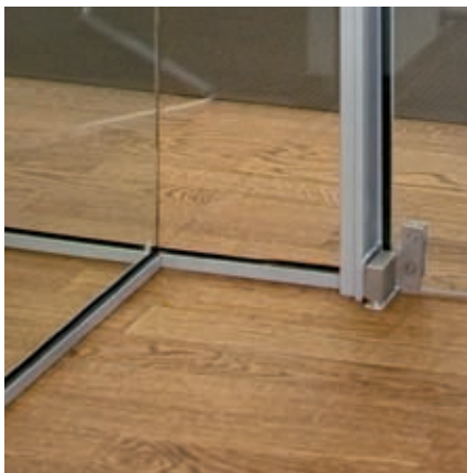
T-joint using silicone seam.
