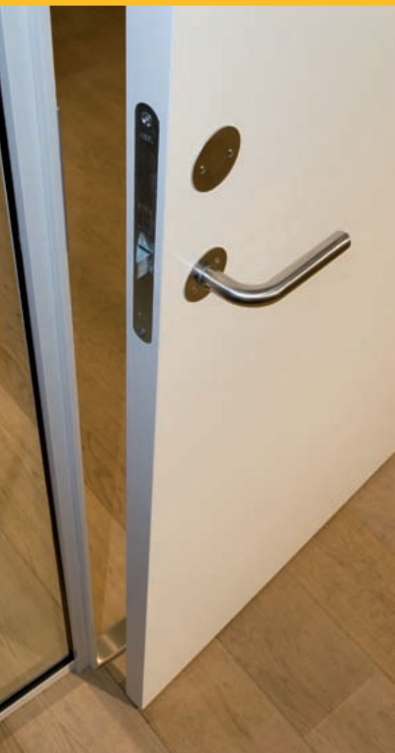
Joint along door frame.
