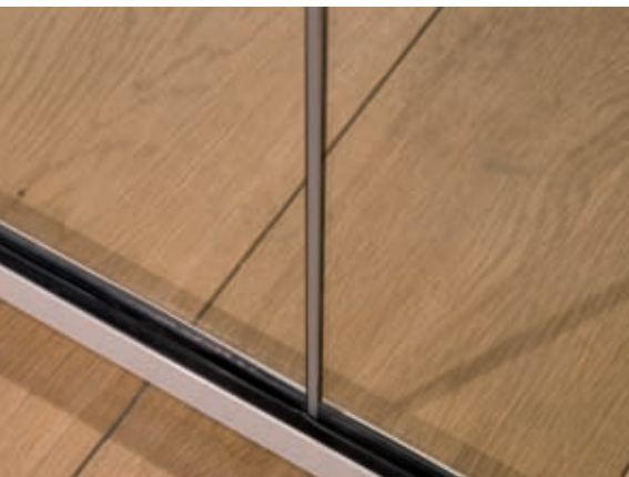
Triplan's silicone seam.
