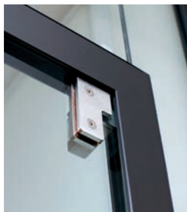
Stainless steel Triplan hinge. Glass door.
