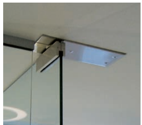
Pivot-hinged glass door with door closer.
