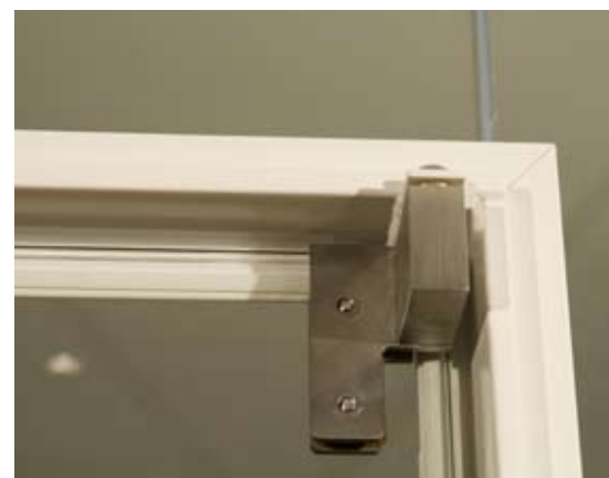
Triplan hinge in stainless steel. Glass door.
