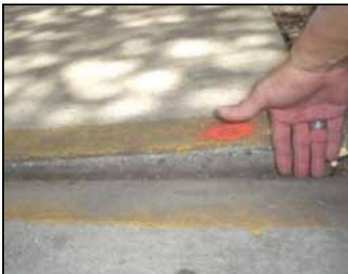
**AFTER: By grinding down the sidewalk, the risk of a trip and fall is greatly reduced.**
