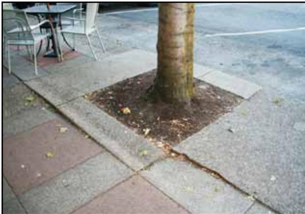
**Raised concrete, pavers, and bricks create a trip hazard. Tree roots can raise sidewalks and walkways when a tree is planted too close.**
