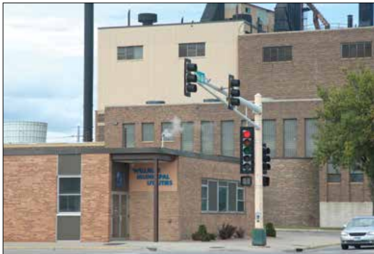
WMU's main downtown location includes offices and a steam cogeneration plant.
