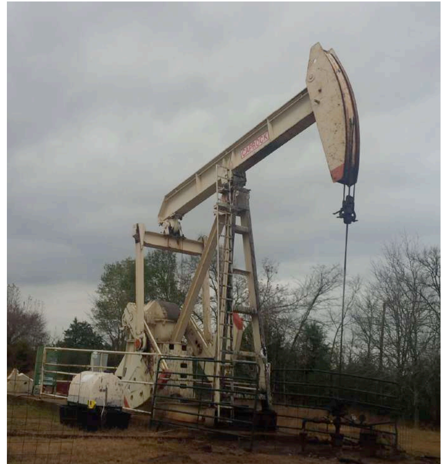
Pump jack at Pine Mills
