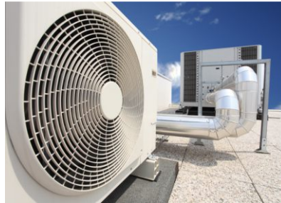
Make-Up Air: Odors & Bio-Chemical Contamination
