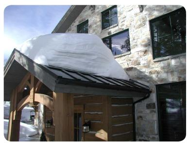
Engineered Roof Deicing' heated T-Panels stop ice buildup on the full length overhang, where it can do the most damage.
