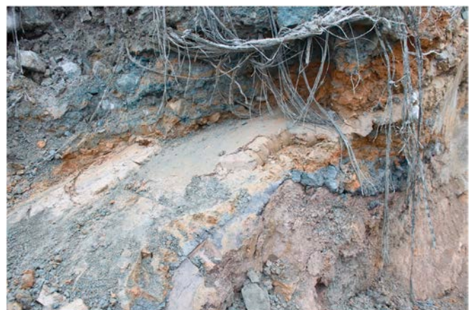
Fig. 2. Example of shear failure plane identified in the trenches excavated below the base of the RSS. (Photo credit: James G. Collin).
