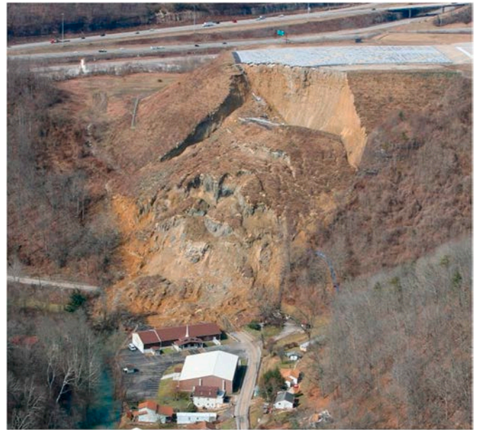
Fig. 6. Aerial failure photo, prior to debris mass creeping over and destroying the church. (Photo credit: W.VA. National Guard).
