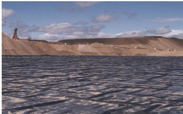
Fig. 4. Example of geomembrane wrinkles in two perpendicular directions [Photo J.P. Giroud].
