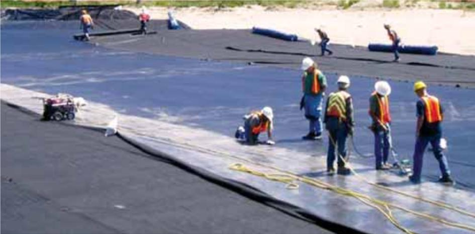
**Photo 8** | Geotextile was deployed over a PVC panel while the panel is welded.
