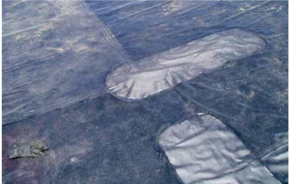
**Photo 6** | Two examples of patches for destructive samples.
