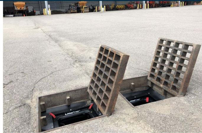
**Enviropod™ Filter** is a high performance catch basin insert that captures and retains sediment, nutrients, heavy metals, litter and debris before they enter the stormwater system.
