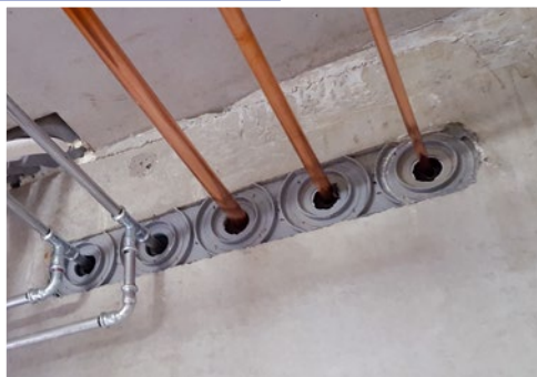
Module penetration units in a concrete wall
