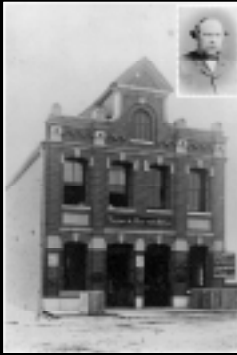
Samuel Yates (ca. 1865), above, and the original structure of 1252 Wharf Street, 1882
