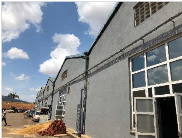
Design Hub/Women's Workshop, Energy Save Installation in Kampala, Uganda - 2019
