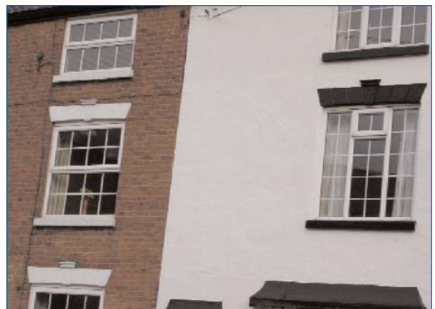
Windows with stone lintels and sills. Window lintels featured have raised keystones
