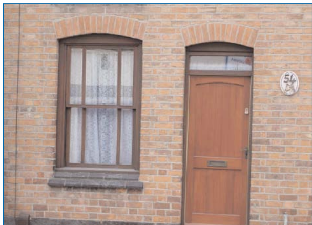
Decorative brick arches (over windows and doors) and brick sills
