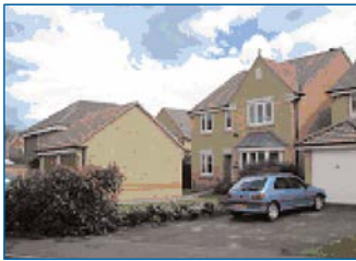
Poorly positioned detached garage
