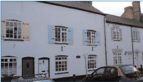
Cottages with inappropriate window shutters
