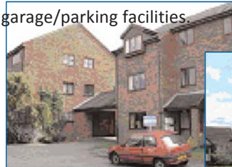
Flats in Willow Close off Pyeharps Road
