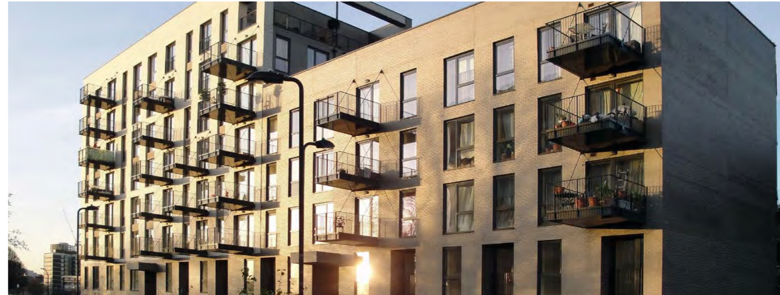
Bridport House, Hackney, London Borough of Hackney
