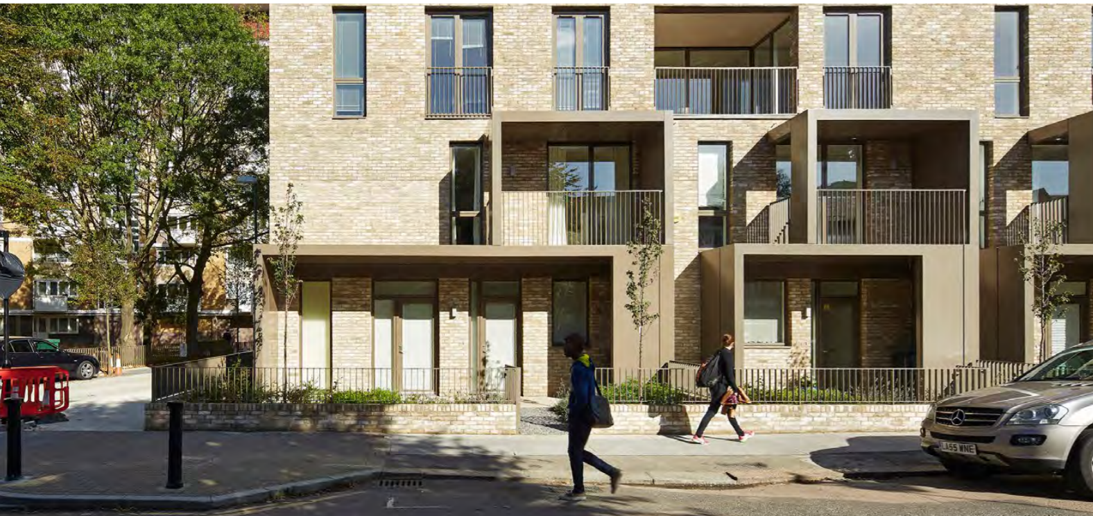
Ely Court, South Kilburn, Catalyst and London Borough of Brent
